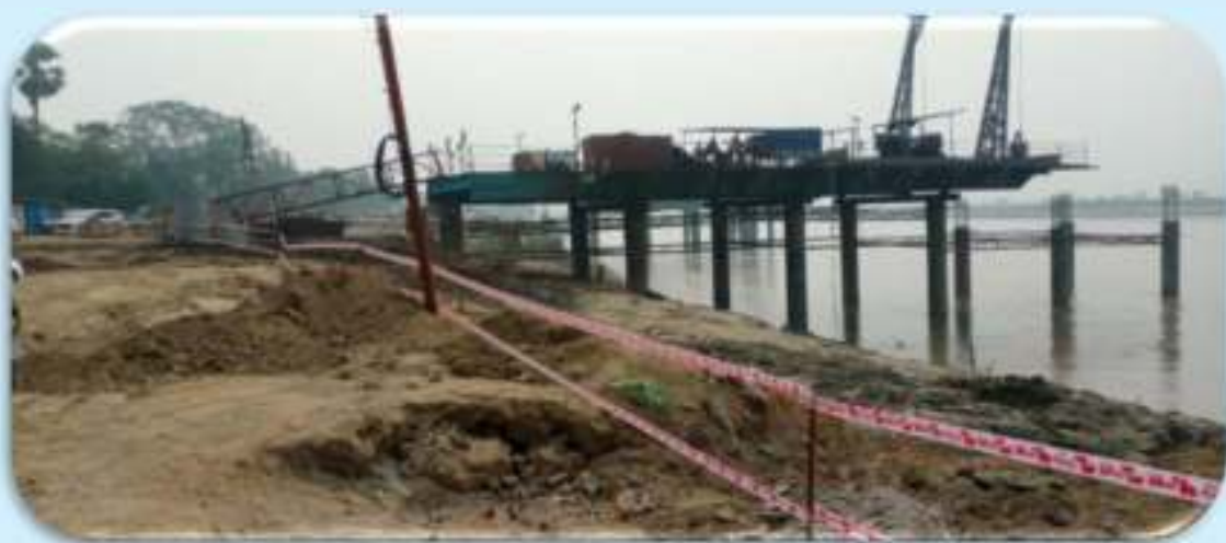
Intermodal terminal at Kalughat
