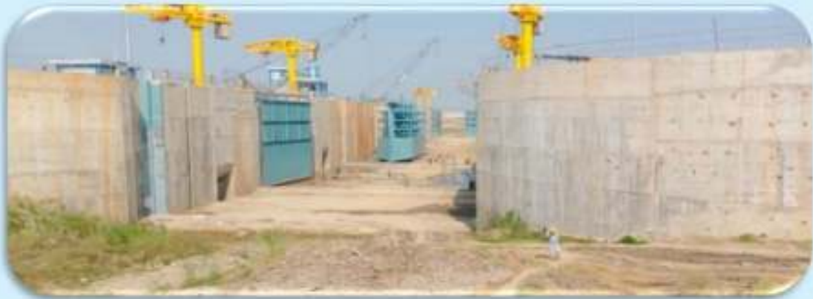
Navigational Lock at Farakka
