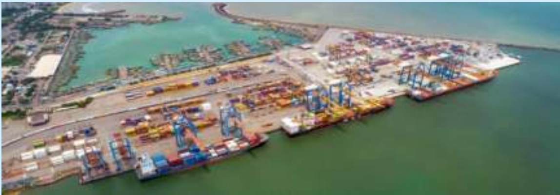
Extension of existing container terminal at Visakhapatnam Port
